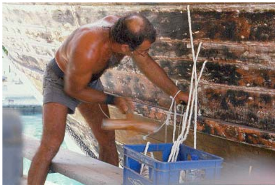
Figure 5. Process of lateral plank caulking of moored vessel
